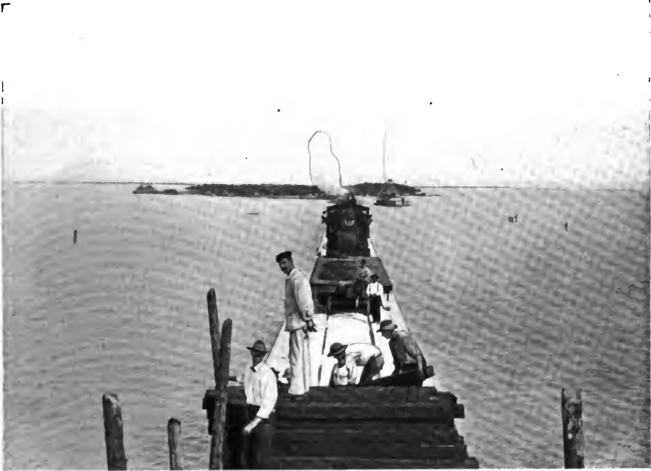
Work train on Long Key Viaduct, Long Key in the distance.
